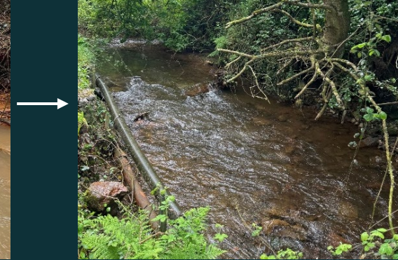
Six months following start of dewatering
