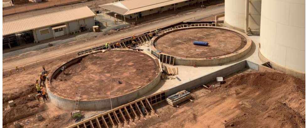
Package 4: Additional leach tank concrete base
