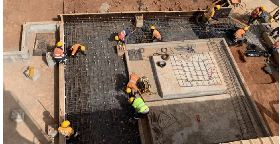
Package 4: Additional leach tank concrete base
